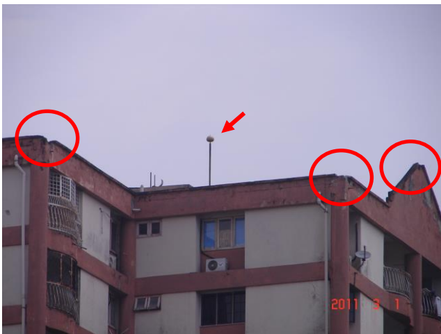
Figure 16. Close-up photograph of an ESE air terminal surrounded by 3 nearby bypasses.
