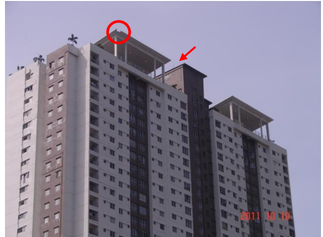
Figure 12. A high-rise building photographed with a bypass about 25 m from an ESE air terminal.
