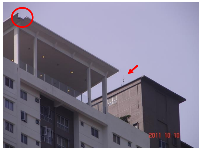
Figure 13. Close-up photograph of the bypass and the ESE air terminal.
